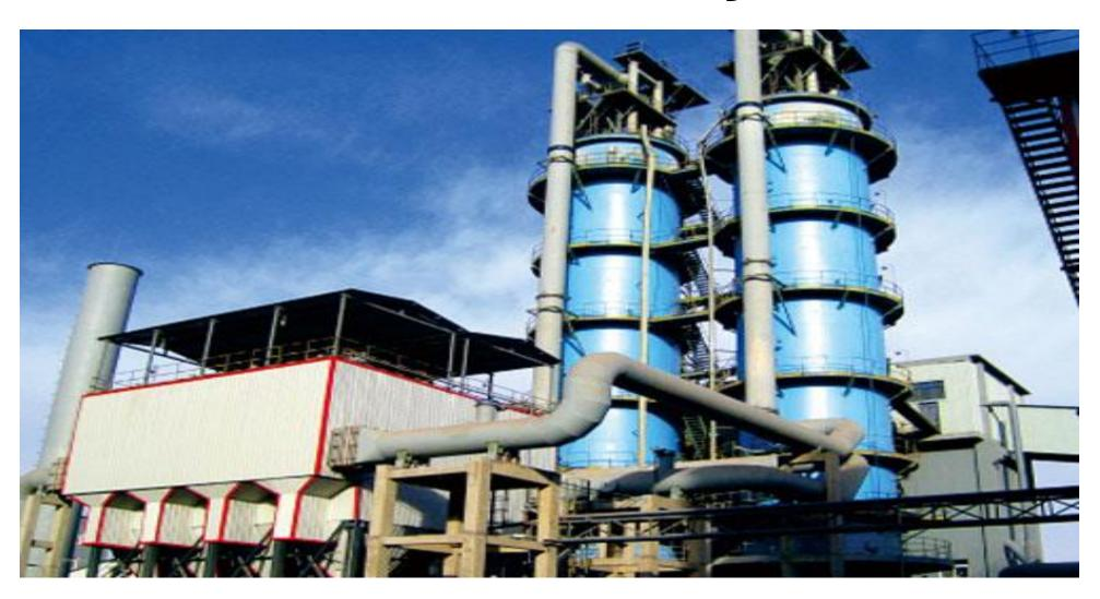
A lime kiln produces quicklime when limestone is calcinated. To achieve this the rotary kiln must reach a temperature upwards of over 1000°C. Refractory bricks are designed to reduce thermal losses and the consumption of energy. Kiln lining refractories improve insulation, reduce maintenance costs, and improve safety while keeping downtime to a minimum.
